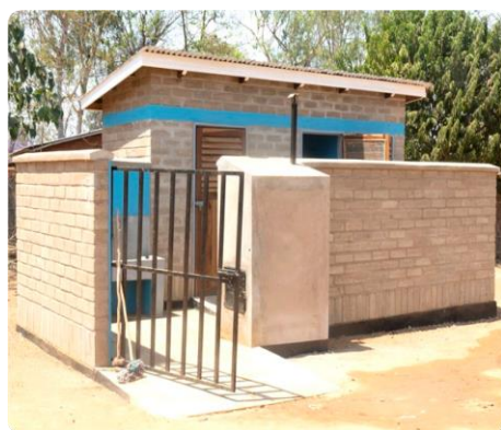
Figure 98: Newly Constructed toilet and shower at Chikwewo Health Care Facility - Machinga
