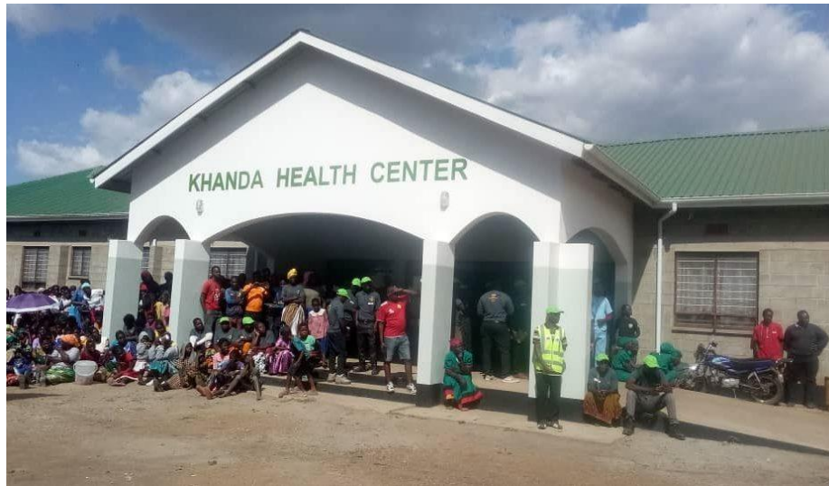
Figure 12: Khanda Health Center, constructed by Village in Partnership.
